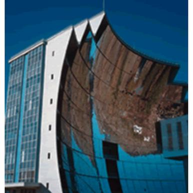
Built in 1969, one side of this building in Odeillo, France, is a large parabolic mirror that focuses sunlight on the building's solar-powered furnace.
