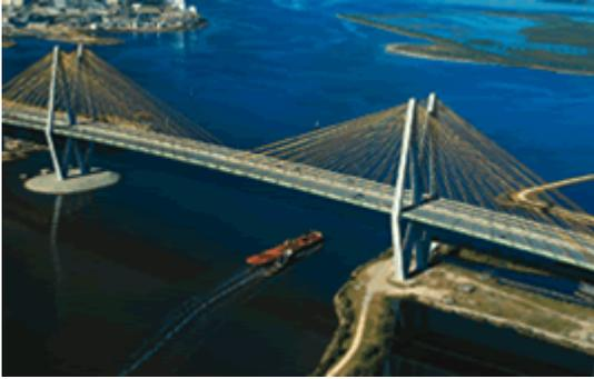
This cable-stay bridge, the Fred Hartman Bridge, connects Baytown, Texas, and La Porte, Texas. Taut cables stretch from the tops of two towers to support the roadway. For more information on cable-stay bridges, see the links at [www.keymath.com/DAA](http://www.keymath.com/DAA).
